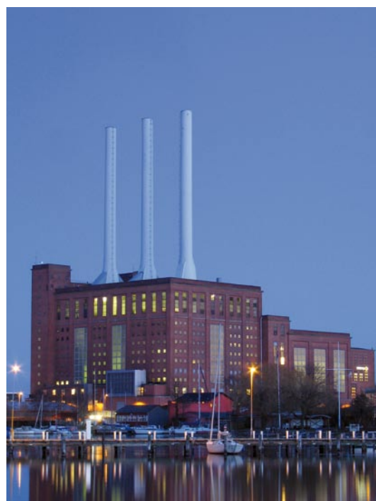
Svanemølle Værket, Copenhagen with two SteamGen™ 4 (pic. DONG Energy)
