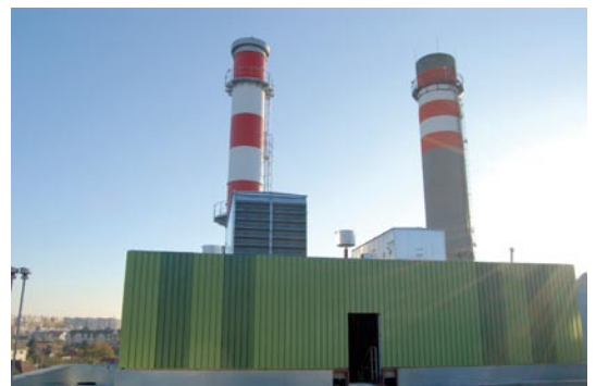
SteamGen™ 6 at Nykce Power plant, Hungary
