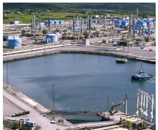
SteamGen™ 6 at Statoil Kårstø Gassprosesseringsanlegg (Pic. Statoil.)
